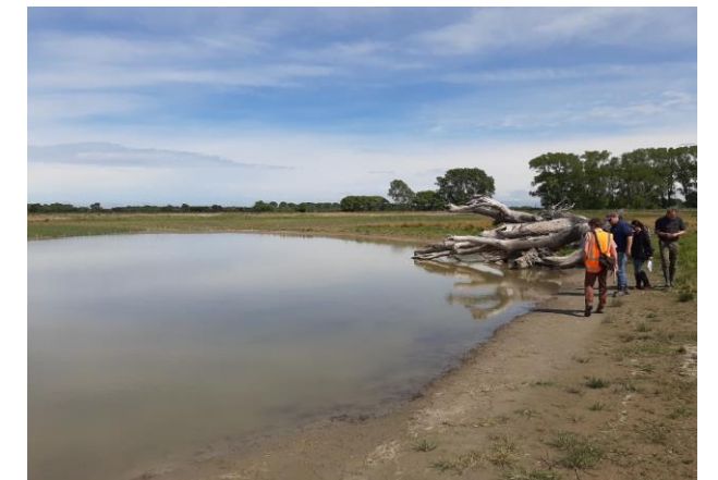
Figure 7. Final inspection of the engineering and earthworks.
