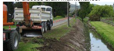
Photo 6: Re-battering Quaifes Road drain.
