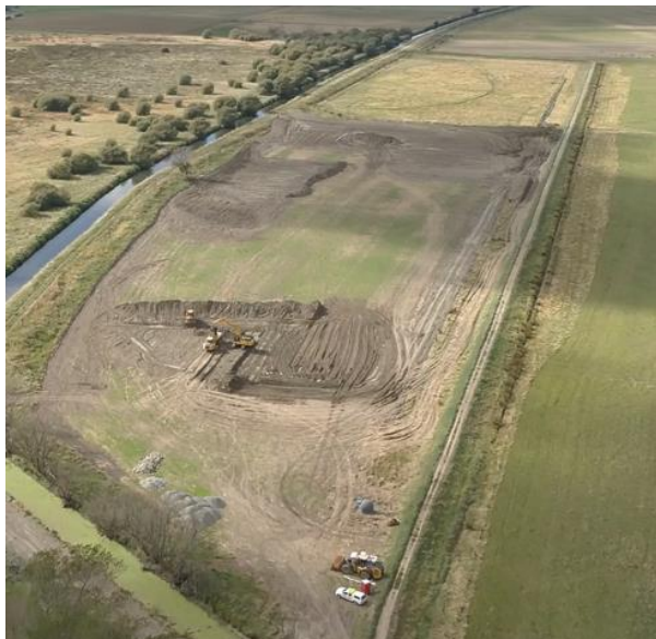
Photo 1: Earthmoving machinery creating the wetland.
