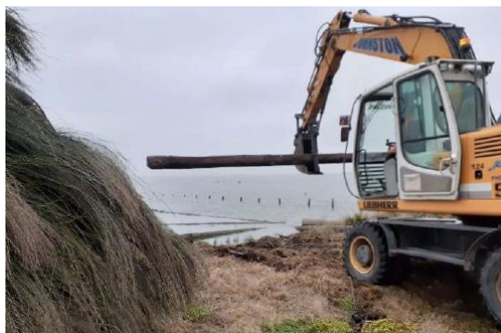
Figure 5. Decoupled logs being lifted ashore.
