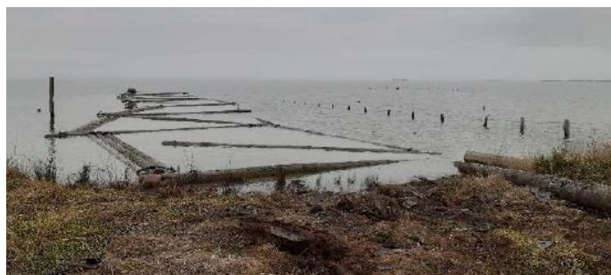
Figure 4. The wave barrier being winched ashore.
