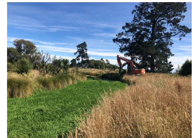
Figure 7. A digger clearing water-weed from Murray's Drain.
